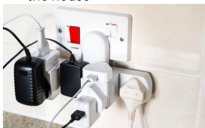
Overloaded plug sockets
