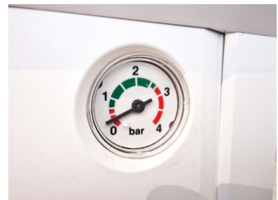
Boiler Pressure low & not between 1-2
