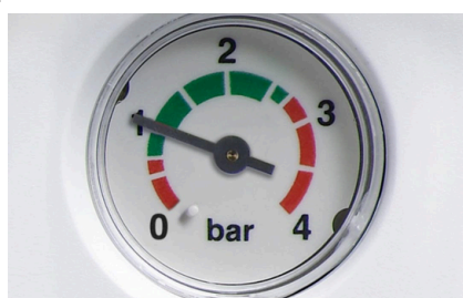
Pressure at 1 on boiler
