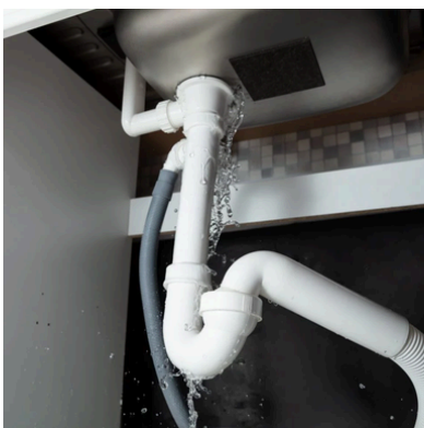
Leak in the sink drain pipes
